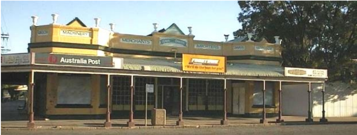
Photo 4: Photo prior to fire in 2002 of Knox and Downs building (Source: Elizabeth Vines 2019)
