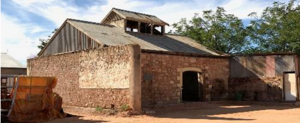
Photo 2: Rear stone building (Source: Elizabeth Vines 2019)
