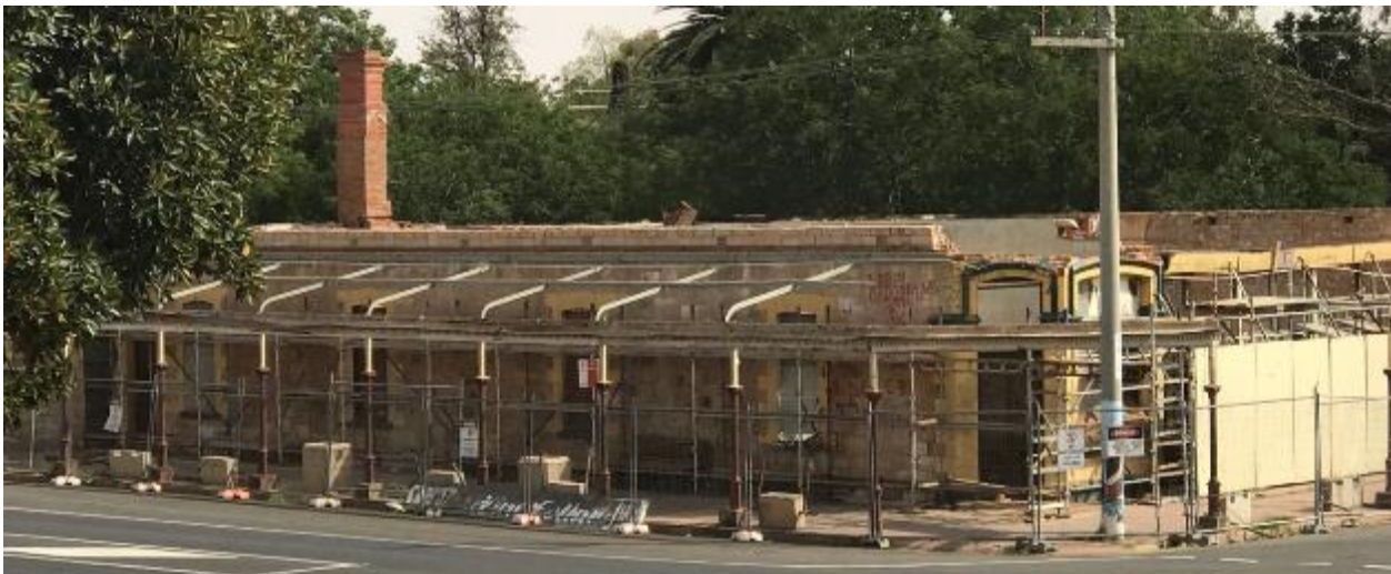
Photo 1: Current condition of building in 2019 (Source: Elizabeth Vines 2019)
