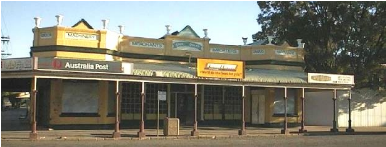
Photo 4: Photo prior to fire in 2002 of Knox and Downs building (Source: Elizabeth Vines 2019)
