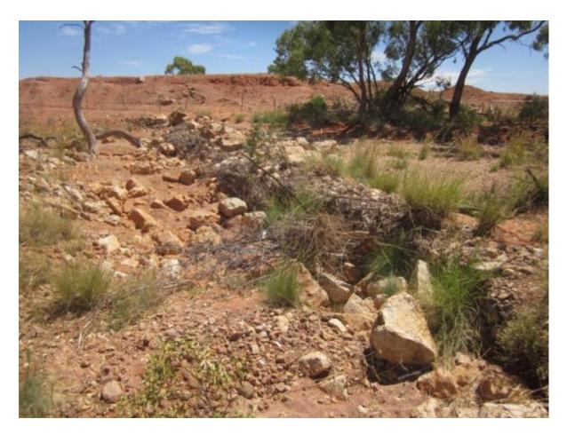
**PLATE 9:** View looking west showing the existing weir, which is a rock-filled gabion structure. The gabion mesh is mostly damaged. The Dam No.3 (Wakefield) embankment is visible in the background of the photo.
