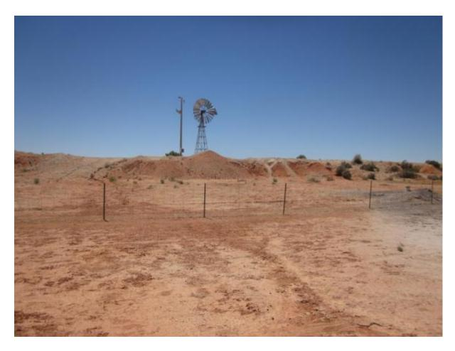
**PLATE 21:** View looking north-east towards Dam No. 3. Some rutting and gullies are visible where water has overflowed the dam embankment.
