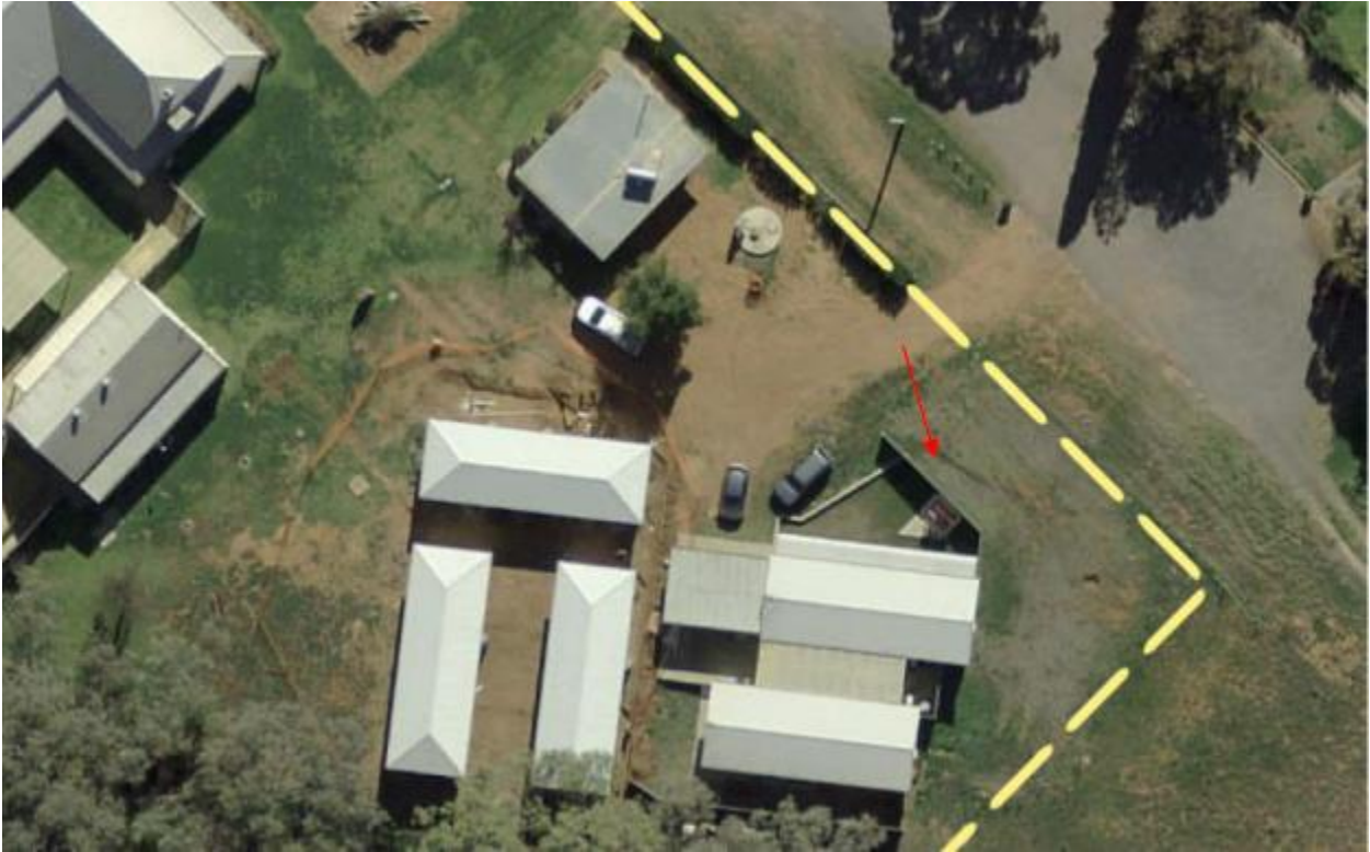
Photo: aerial photo of site at 5-19 Wilson Street Wilcannia May 2021 with nominated site of antennae (Source: 6 maps 2021)
