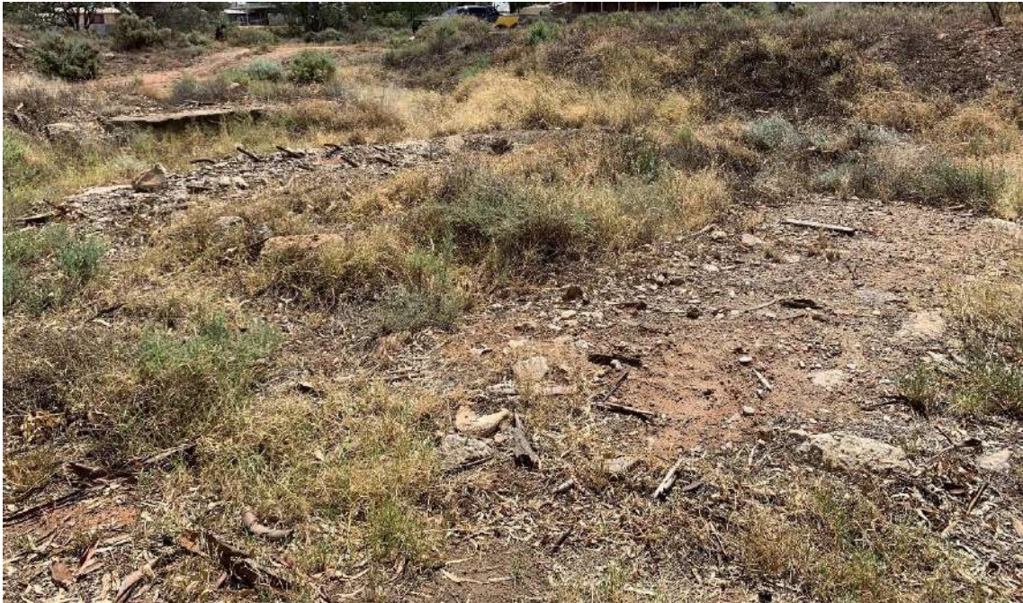
Figure 2.6: Photo D – Remnants of old building adjacent pump shed.
