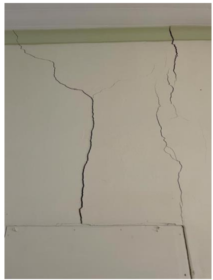
Internal views showing typical cracks to floor (LHS) and walls (centre and right)
