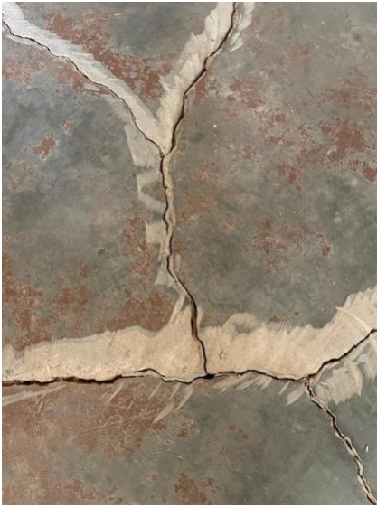
Internal views showing typical cracks to floor (LHS) and walls (centre and right)
