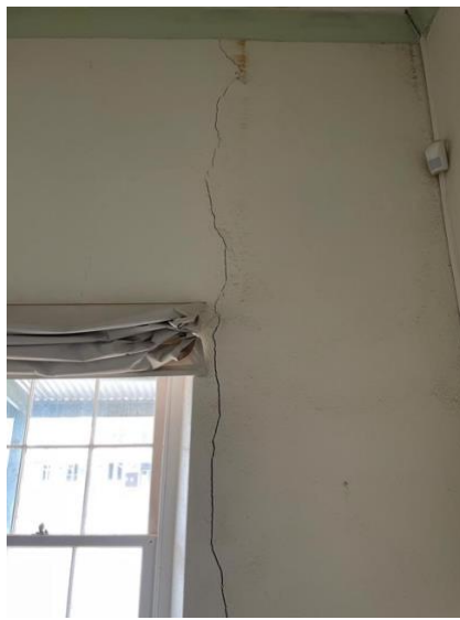
Internal views showing typical cracks to floor (LHS) and walls (centre and right)
