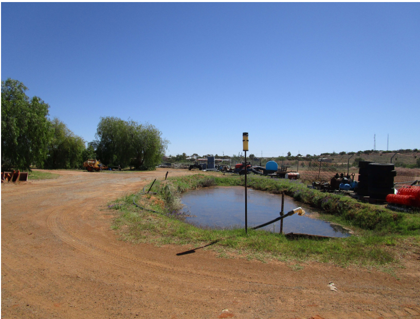
Figure 2-5 View of the existing WTP site, looking north.
