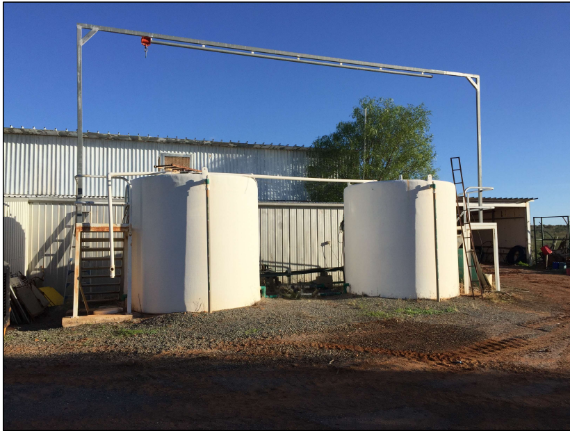
Figure 2-4 View of the existing WTP building and storage tanks at the site.
