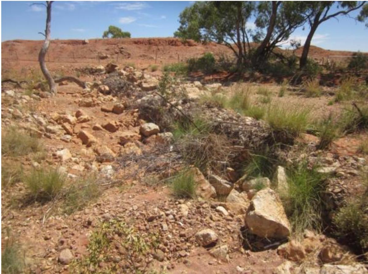
**PLATE 9:** View looking west showing the existing weir, which is a rock-filled gabion structure. The gabion mesh is mostly damaged. The Dam No.3 (Wakefield) embankment is visible in the background of the photo.
