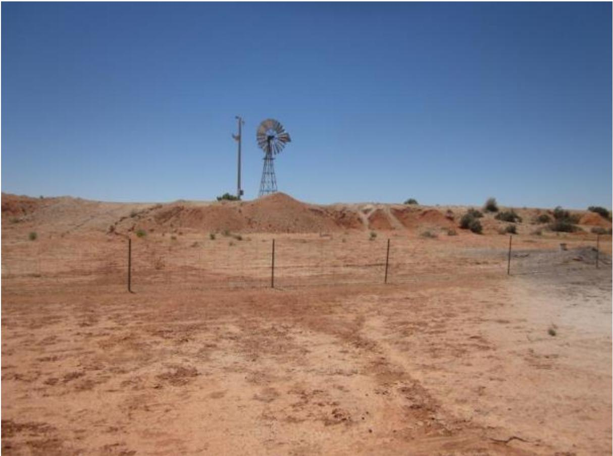
**PLATE 21:** View looking north-east towards Dam No. 3. Some rutting and gullies are visible where water has overflowed the dam embankment.
