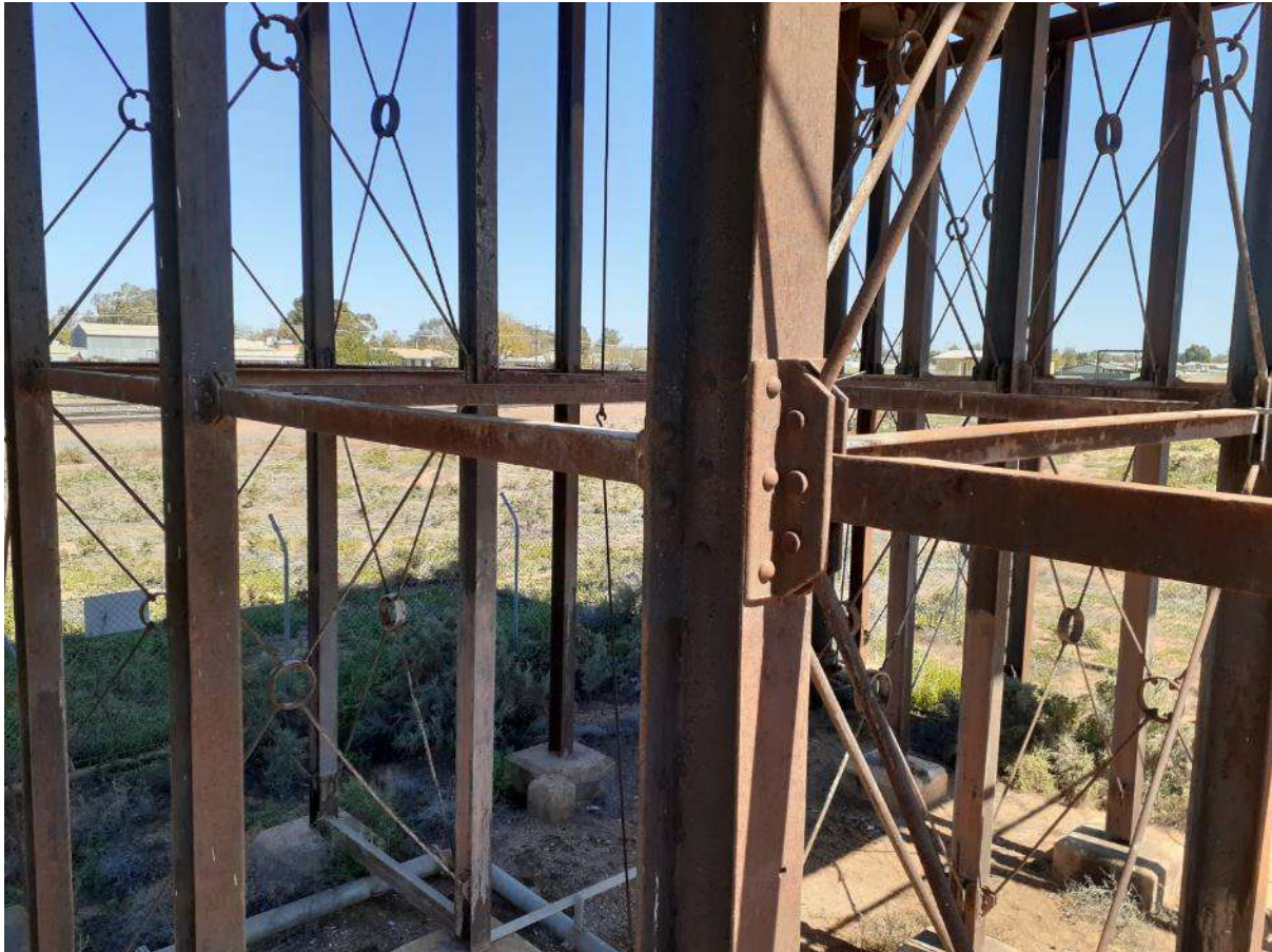
Figure 17 - General condition of structural steelwork - Minor surface rust
