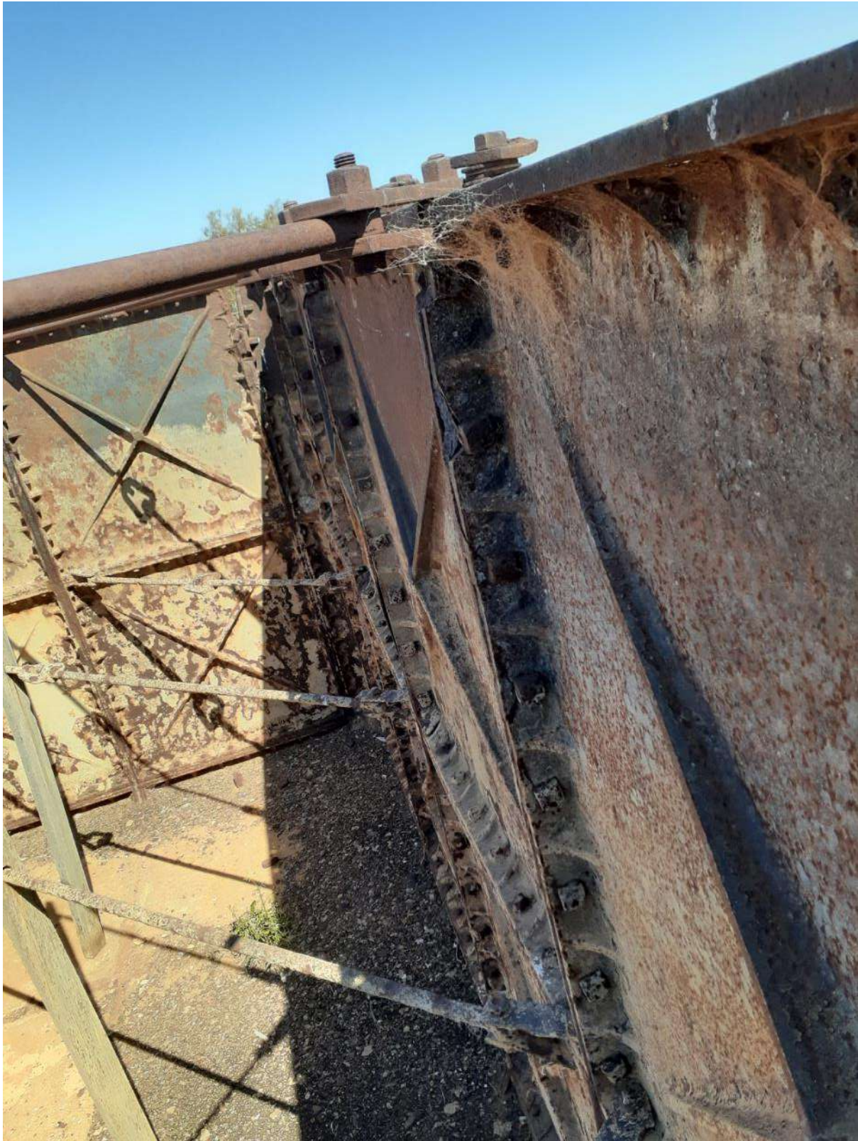
Figure 12 - Typical example of the internal walls - note the frequency of bolt damage.
