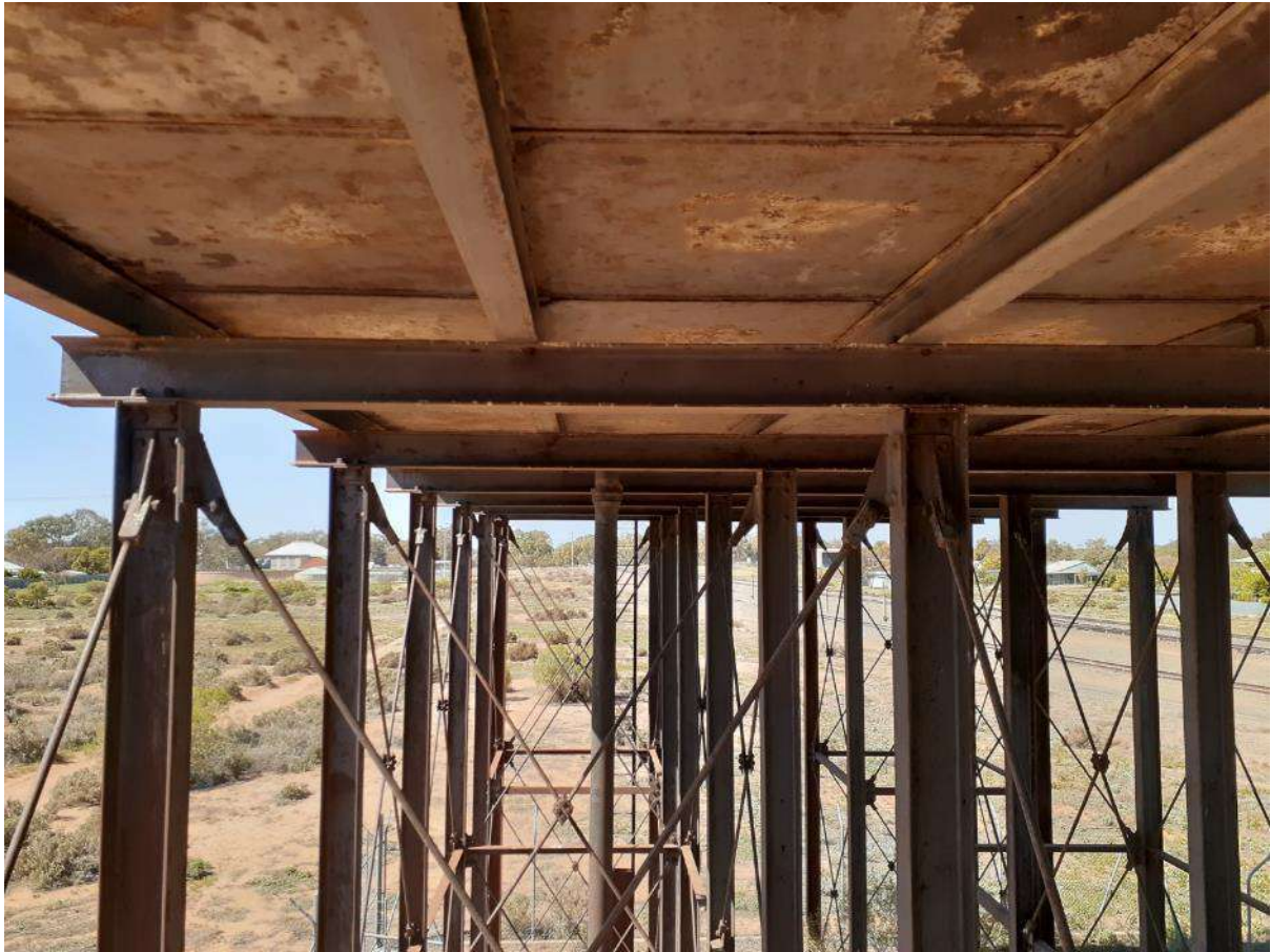
Figure 19 - Typical Joists and Bearers beneath the East and Centre Tanks - Minor surface rust
