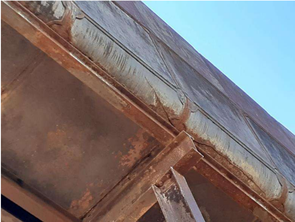
Figure 7 - Further cracking at the interface between the walls & the tank floor
