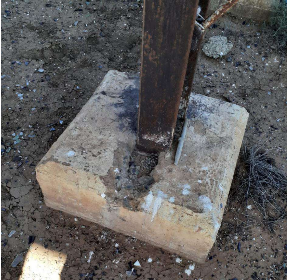
Figure 16 - Breakout on Plinth, West Tank
