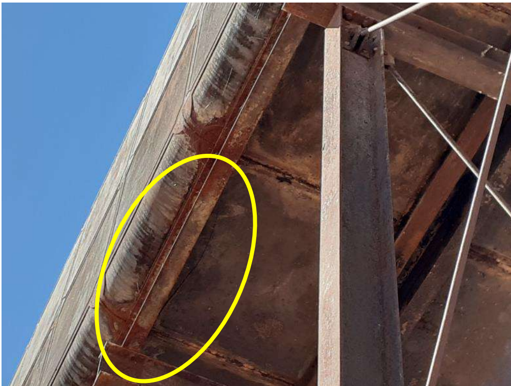
Figure 8 – Example of Cracking developing in Cast Iron Floor
