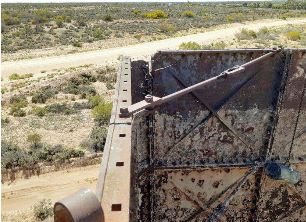
Figure 13 - Further example of deterioration of bolted connections. Some corners are more progressed than others. All corners shown development into this type of deterioration.
