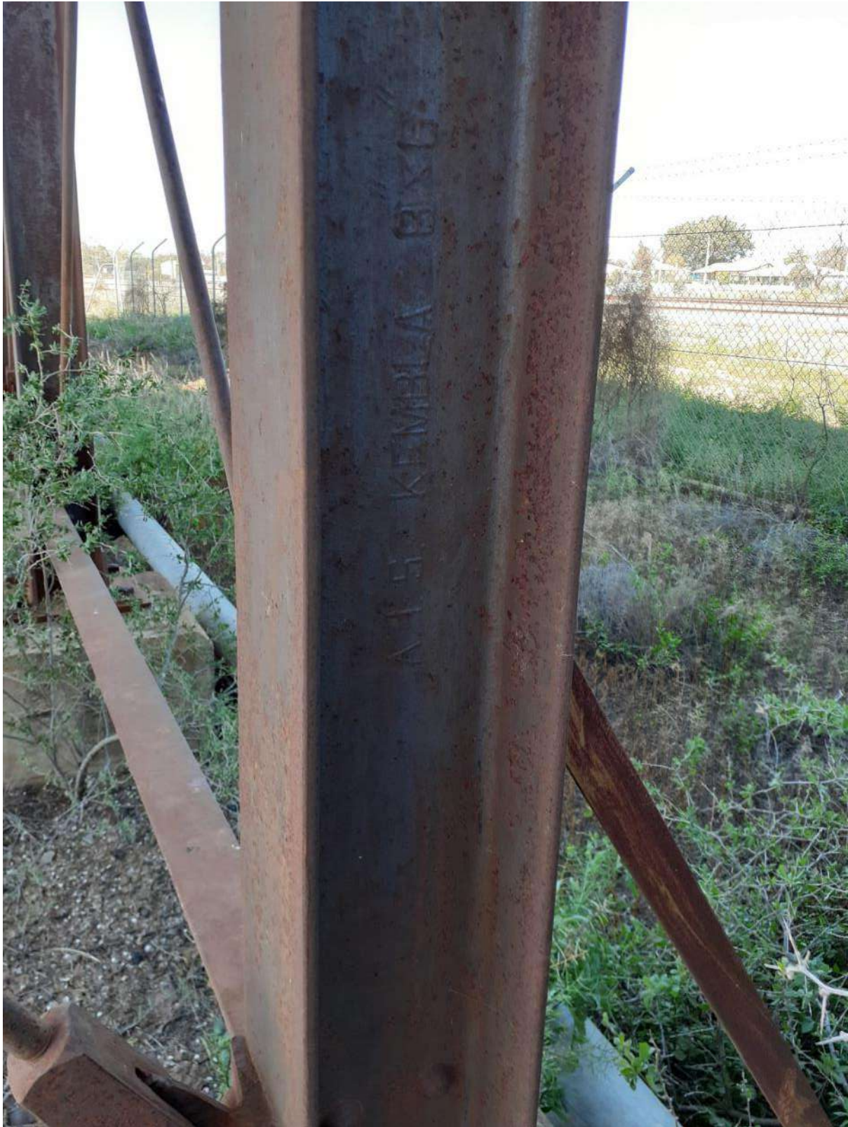
Figure 20 - Typical Column for East & Centre Tanks. Note sparse evidence of previous surface coating.
