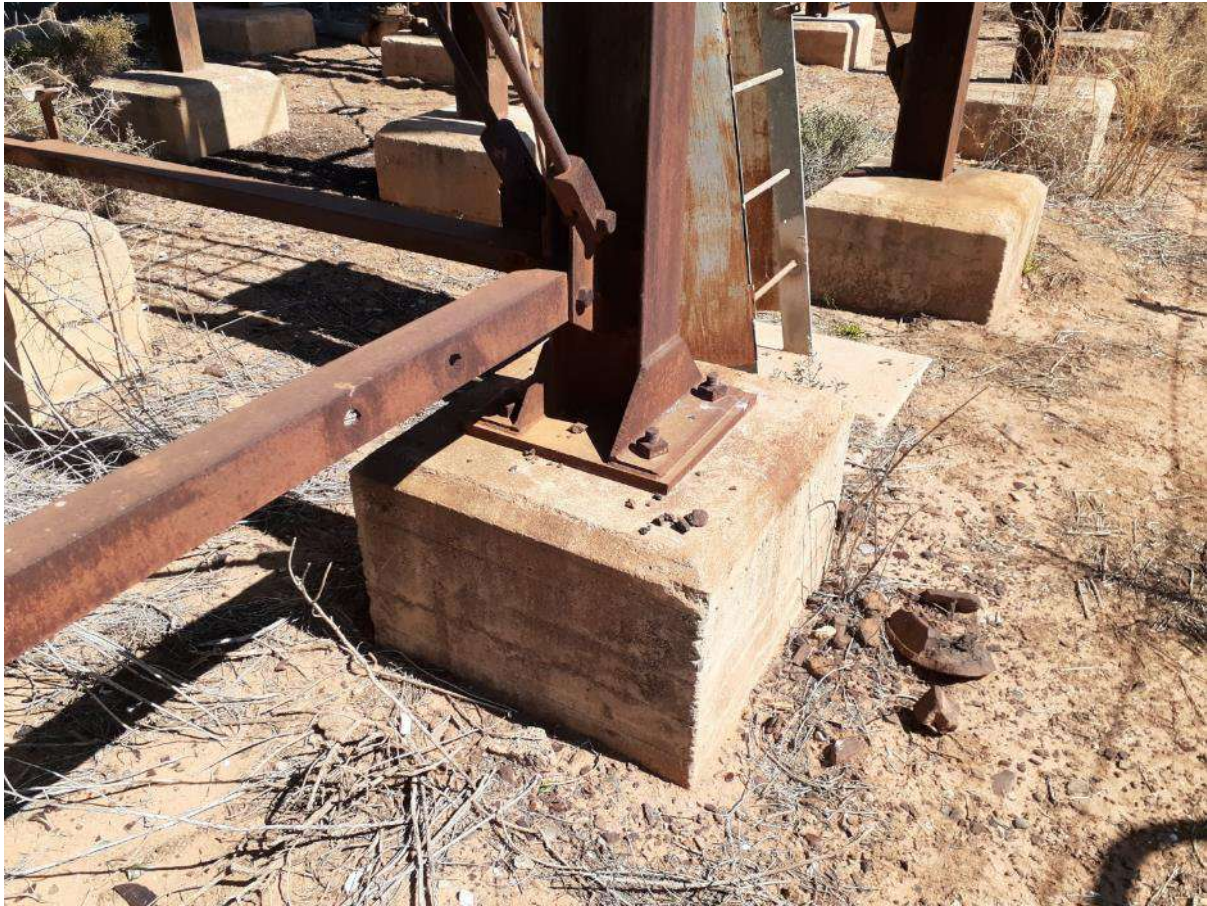
Figure 18 - Minor surface corrosion - Looking West at a plinth on the second tank. Note difference in column connection of the West tank in the background.
