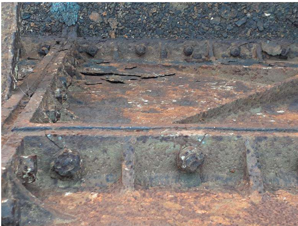
Figure 10 - Cracking developing - Bolts slowly blowing out. Looking from top of tank down to the floor.
