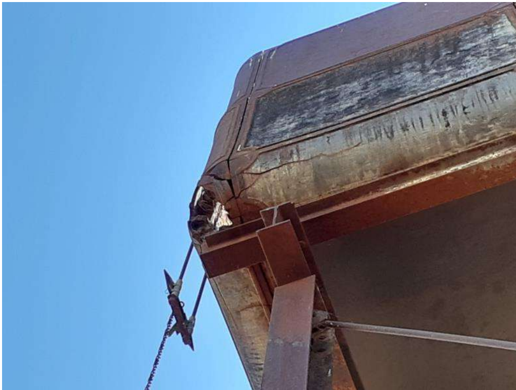
Figure 6 - Example of cracking & failing cast iron. Some corners are more progressed than others.
