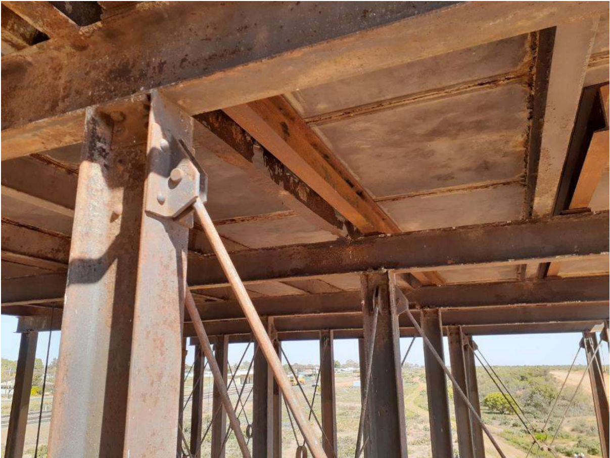
Figure 15 - Example of web of floor joist corroded away. Note second joist installed beside it.
