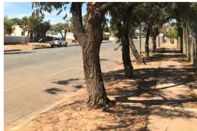
Concrete kerb with concrete footpath in turf
