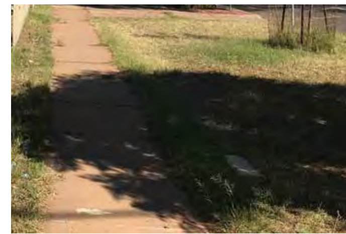
Concrete footpath in turf
