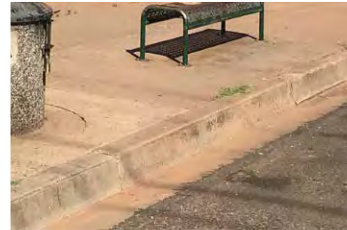
Concrete kerb and footpath
