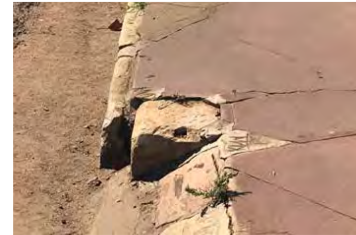
Sandstone Kerb in poor condition
