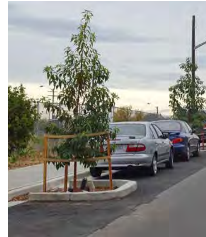
Tree planting to road shoulder Concrete kerb protection
