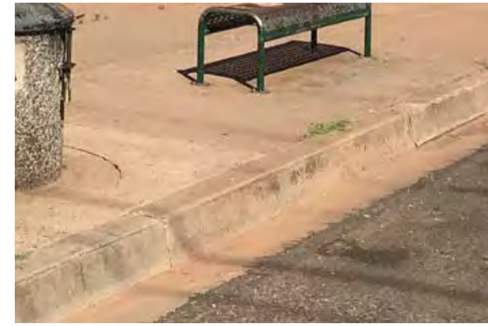
Concrete kerb and footpath
