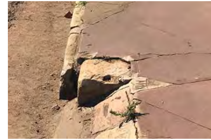
Sandstone Kerb in poor condition
