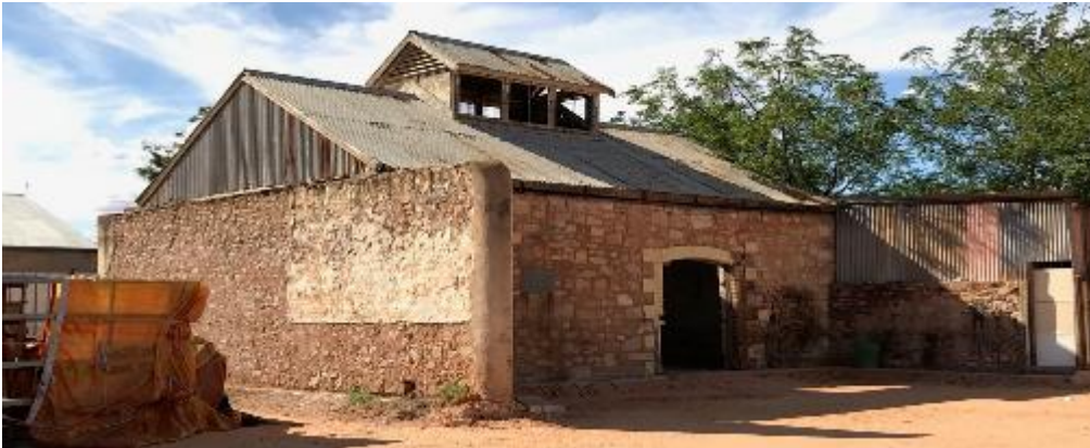
Photo 2: Rear stone building (Source: Elizabeth Vines 2019)
