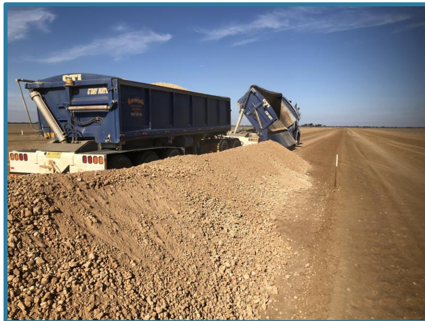
Gravel being tipped on prepared formation, Wool Track
