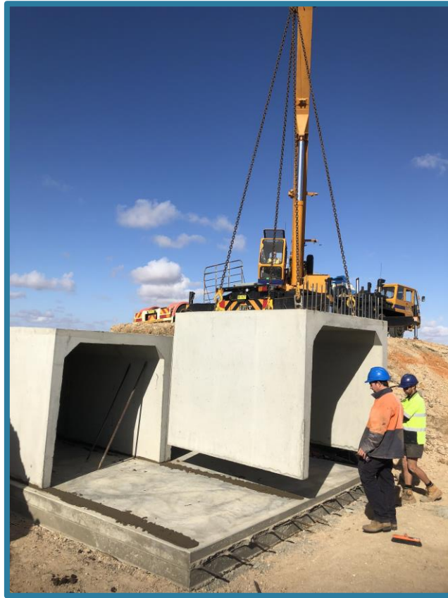
Culverts being placed at Willandra Creek Crossing, Wool Track
