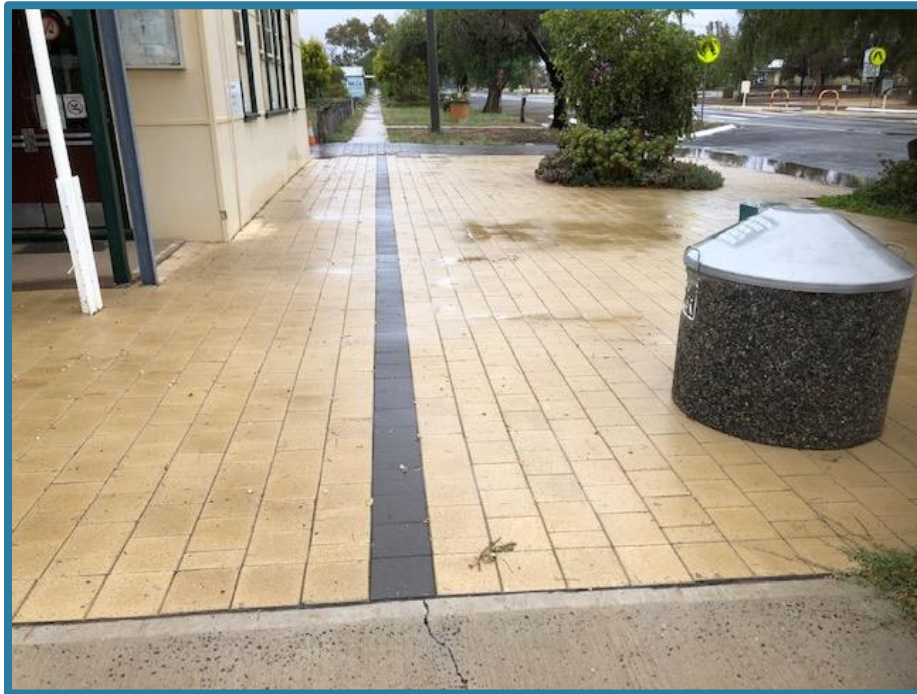
Additional paving area was completed at Ivanhoe, in front of the School
