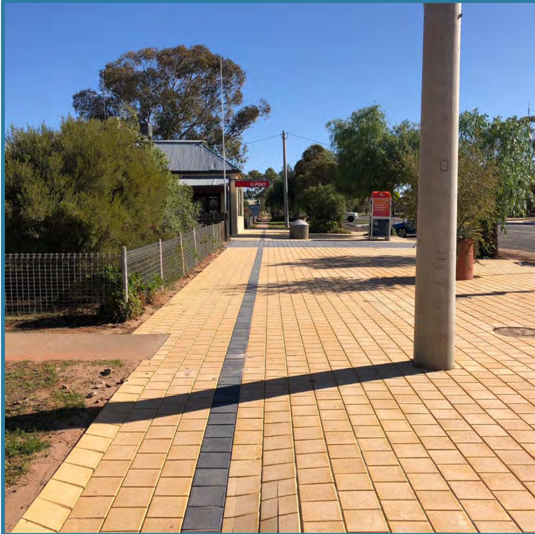
Additional paving area was completed at Ivanhoe, adjacent to the Post Office
