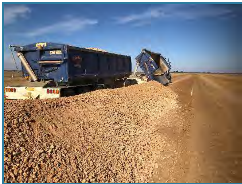
Gravel being tipped on prepared formation, Wool Track
