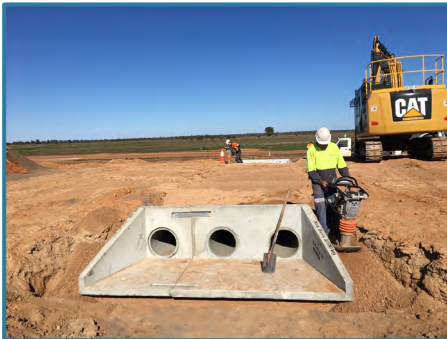
Culvert installation Gypsum Mine North Initial Seal Project, Cobb Highway
