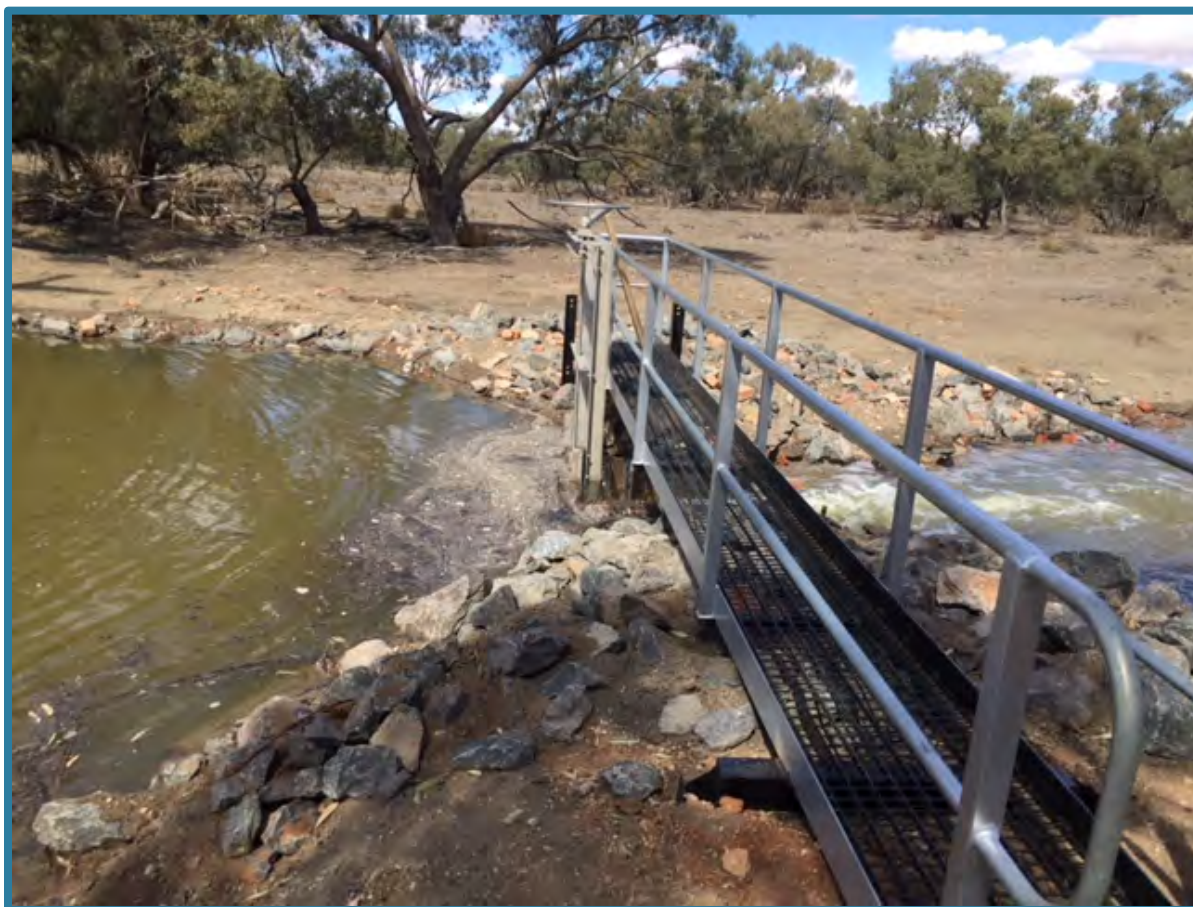
New Weir structure at Ivanhoe's Willandra Creek offtake
