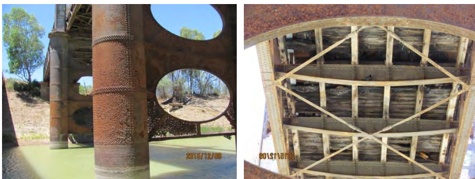
2015 photos of the bridge (Jim Wilson photos)
