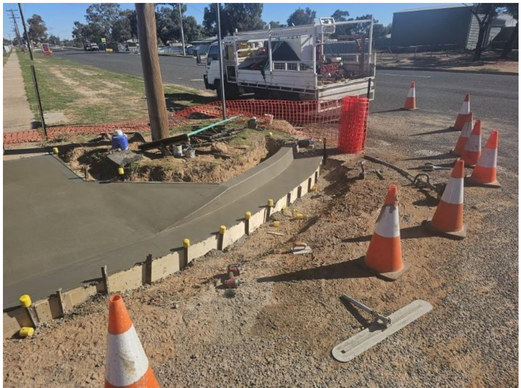
Menindee kerb and pram ramp replacement, Haberfield/ Menindee Street intersection
