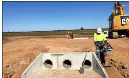
Culvert installation, Initial Seal Project, Cobb Highway.
