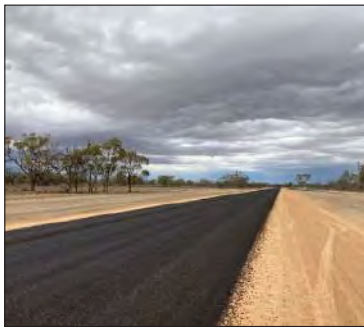
New Seal Section Pooncarie Road.
