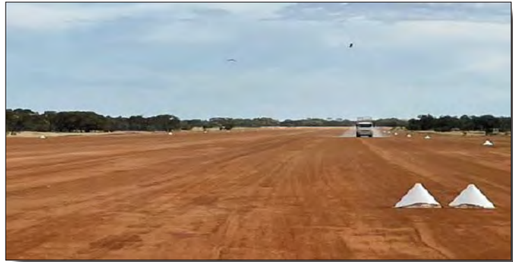
Grading and levelling works, Emmdale Airstrip.
