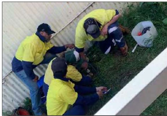
Ivanhoe Team seen here working hard to fix a leak.
