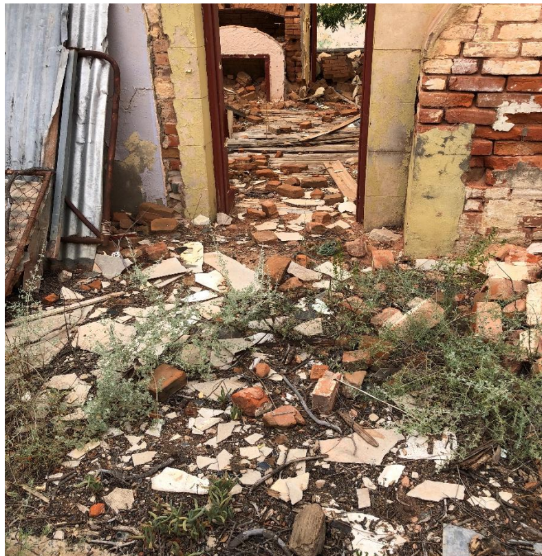
Figure 6.5: Larger pieces of fibre cement near entrance and inside the structure.
