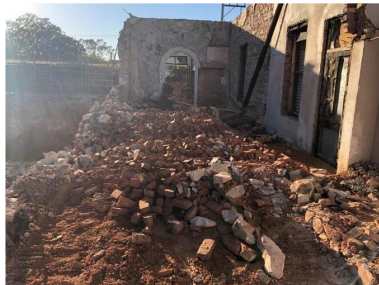
Image 24: During Removal of Contaminated Bricks and Timber Flooring from Rooms between Fireplace Room and West Wing
