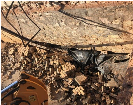
Image 17: During Removal of Front Windows and Demolition of Main Cellar Brick Skin Wall
