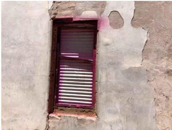
Image 29: Following Removal of Contaminated Bricks and Timber Floor West Wing Room-PVA Spray sealed Timber Windows and Door Frames to be removed at a later date
