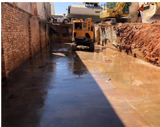
Image 13: At completion of Removal of Materials from the Central Cellar
