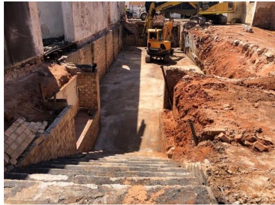
Image 12: Removal of Materials from Central Cellar
