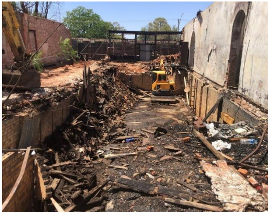
Image 11: During Removal of Main Section Floor and Front Wall
