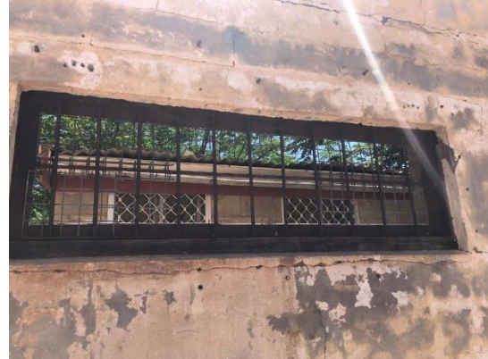
Image 37: Timber at bottom of steel window in North East Corner. To remain in-situ. Has been sprayed with lacquer solution.
