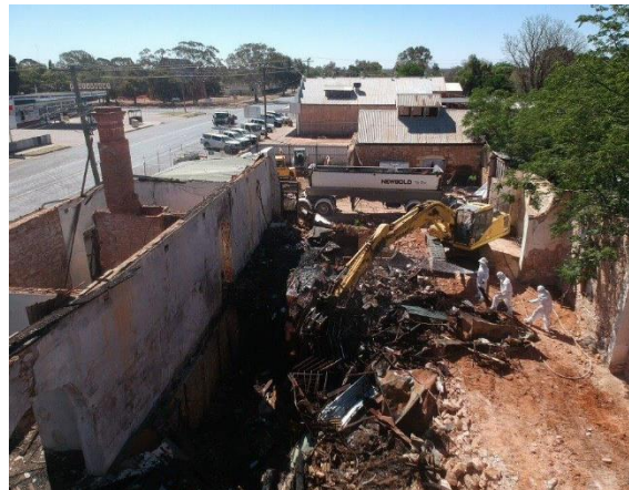
Image 10: During Removal of Main Section Floor and Front Wall
