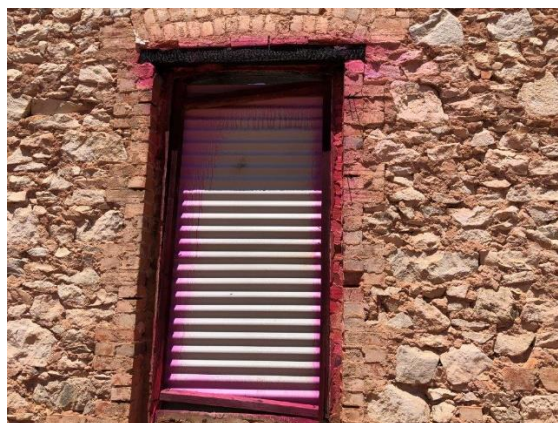
Image 28: Following Removal of Contaminated Bricks and Timber Floor West Wing Room-PVA Spray sealed Timber Windows and Door Frames to be removed at a later date
