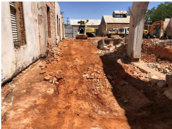
Image 25: Following Removal of Contaminated Bricks and Timber Floor West Wing Room
