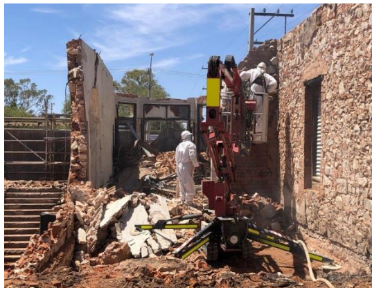
Image 23: During Removal of Contaminated Bricks and Timber Flooring from Rooms between Fireplace Room and West Wing
