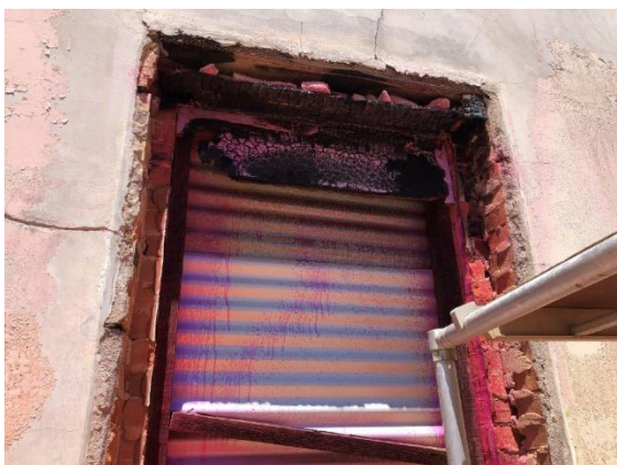
Image 27: Following Removal of Contaminated Bricks and Timber Floor West Wing Room-PVA Spray sealed Timber Windows and Door Frames to be removed at a later date
