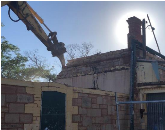
Image 19: During Removal of Roof and Internal wall to Concrete Room
