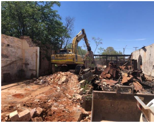
Image 7: Demolition of the North East Section Internal Wall
