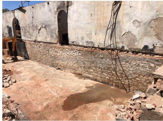
Image 18: At Completion of Removal of Front Windows and Demolition of Main Cellar Brick Skin Wall
