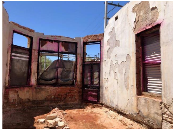
Image 30: Following Removal of Contaminated Bricks and Timber Floor West Wing Room-PVA Spray sealed Timber Windows and Door Frames to be removed at a later date
