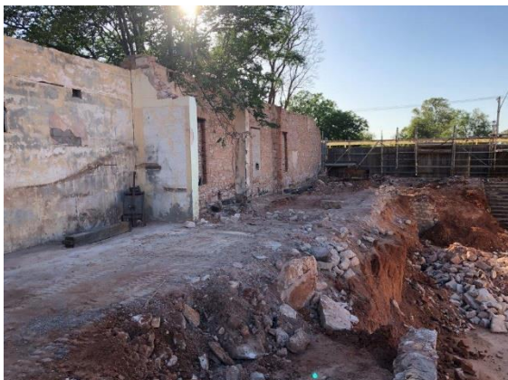
Image 35: Following Removal Subfloor Contamination at North corner of main Cellar in North East Section
