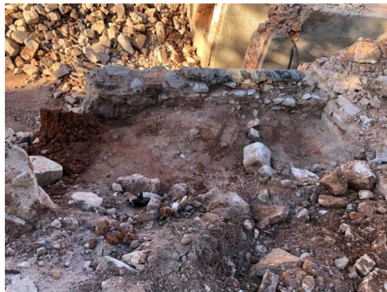
Image 34: Following Removal Subfloor Contamination at North corner of main Cellar in North East Section
