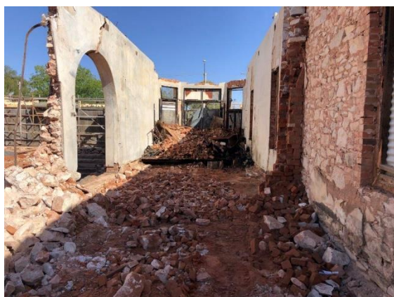
Image 23: At completion of Contaminated Bricks and Timber Flooring from Rooms between Fireplace Room and West Wing
