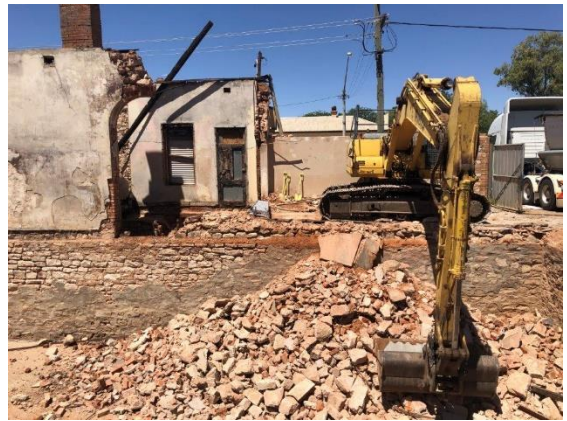
Image 20: Following Removal of Roof and Internal wall to Concrete Room
