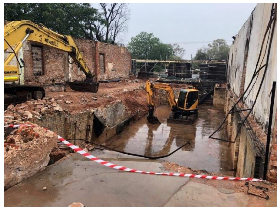
Image 14: At completion of Removal of Materials from the Central Cellar
