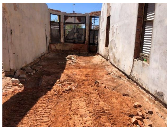
Image 24: Following Removal of Contaminated Bricks and Timber Floor West Wing Room
