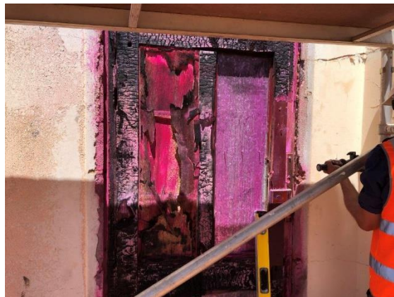
Image 26: Following Removal of Contaminated Bricks and Timber Floor West Wing Room-PVA Spray sealed Timber Windows and Door Frames to be removed at a later date
