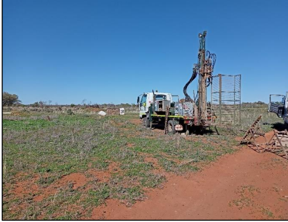
Figure 2: View south towards Bore 4 location
