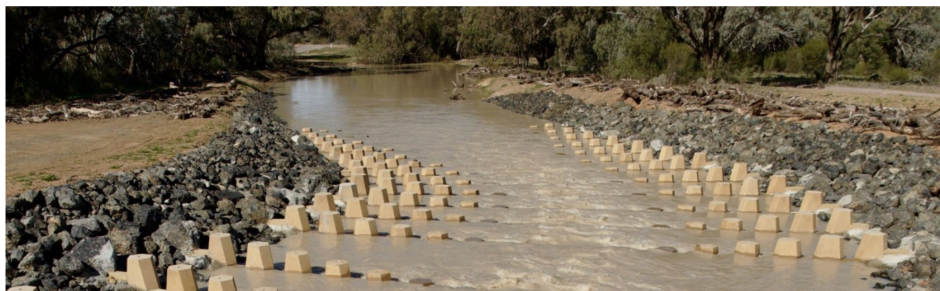
Image of Homestead Dam rock-ramp fishway, Toorale.
