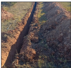
Pictured: Ivanhoe trench works.
