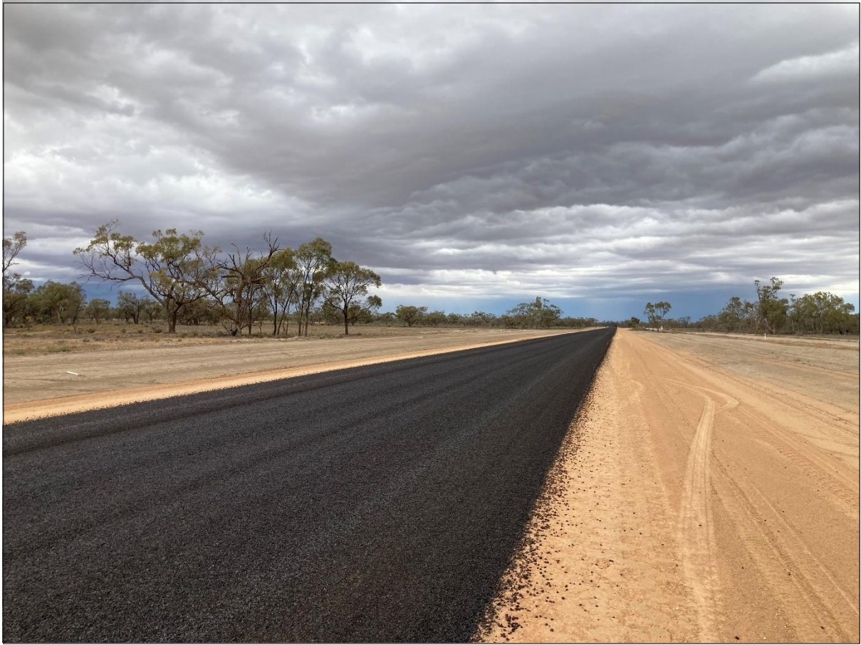
New Seal Section, Pooncarie Road
