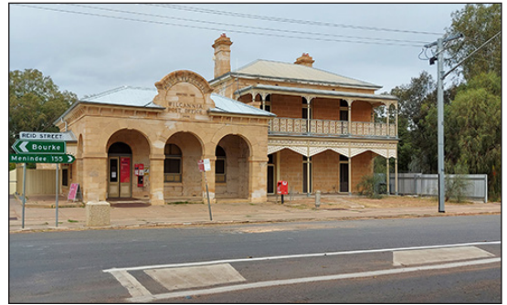
Wilcannia Post Office Building.
