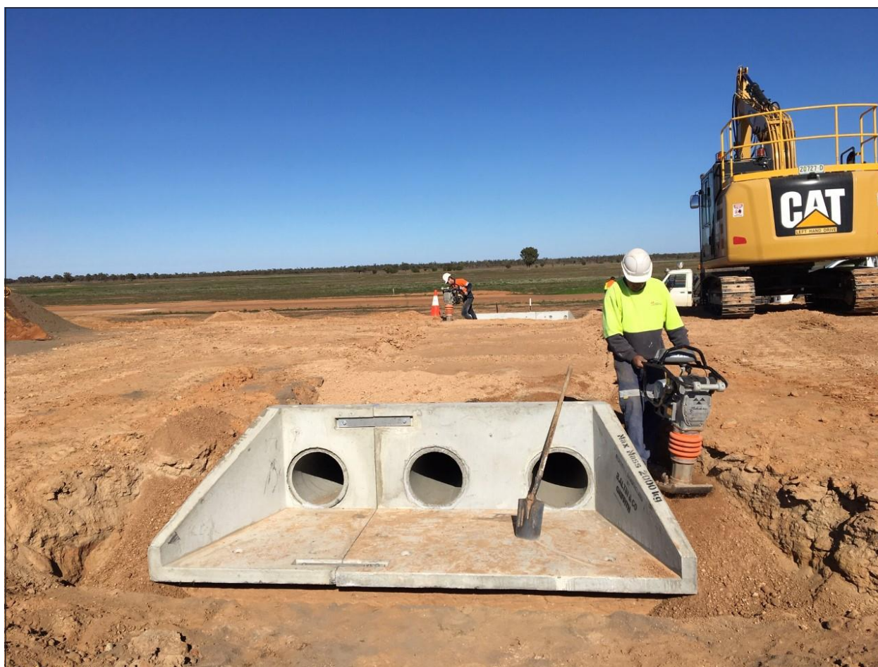
Culvert installation Rosewood South Initial Seal Project, Cobb Highway
