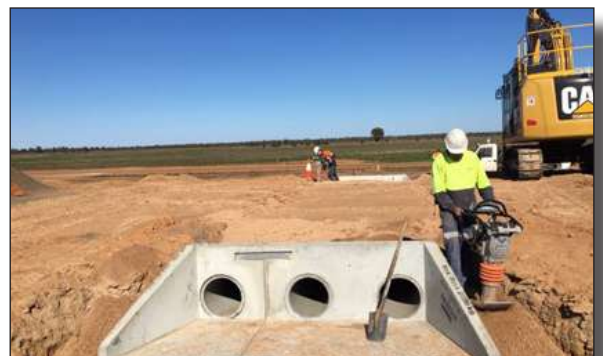
Culvert installation, Initial Seal Project, Cobb Highway.
